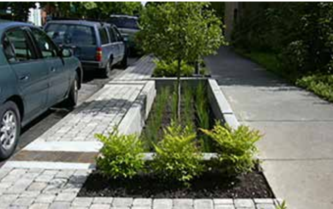
Bio-filtration in Sidewalk Area
