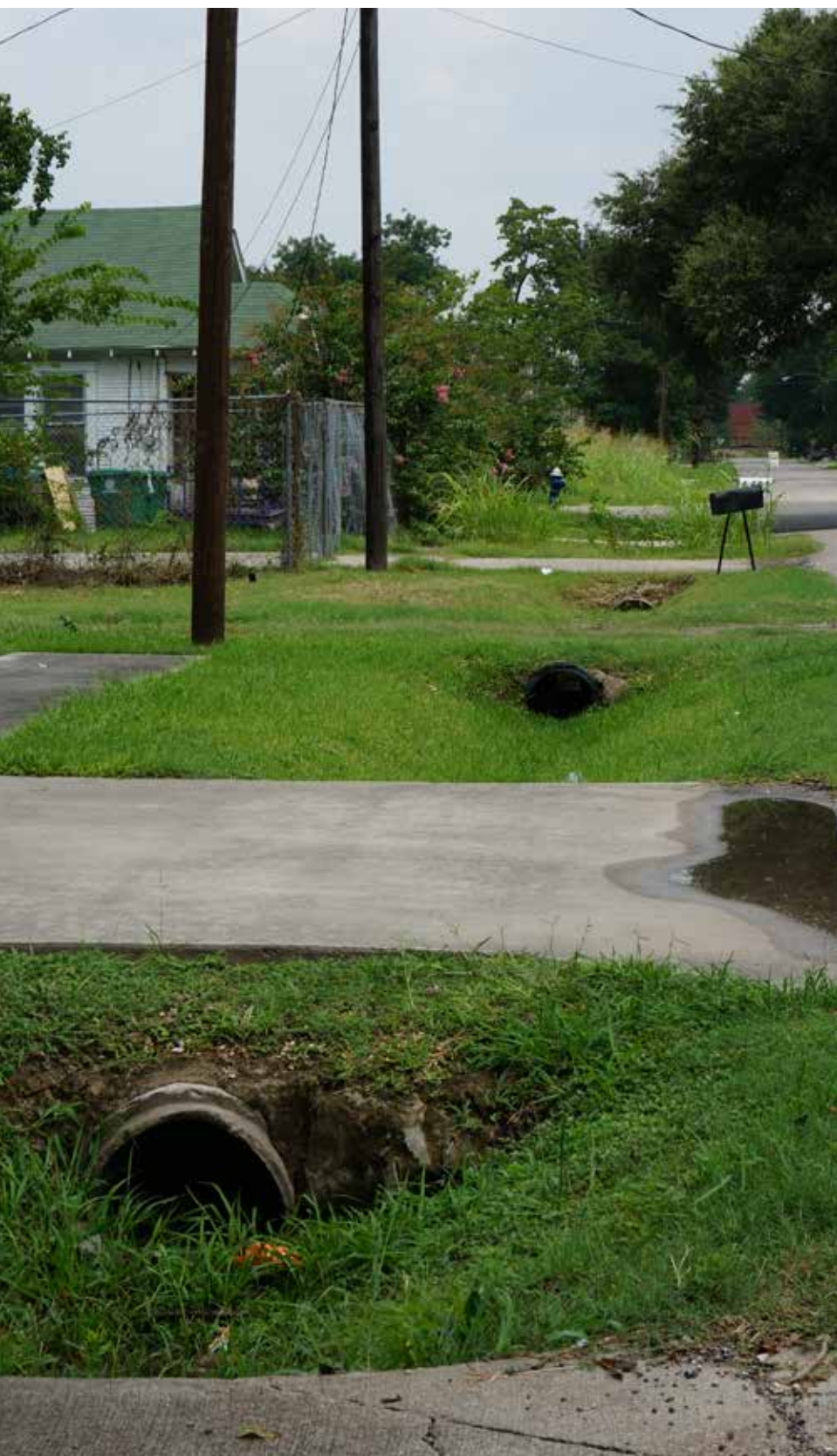
Common storm water management technique used within Houston neighborhoods, to collect water in drainage ditches
